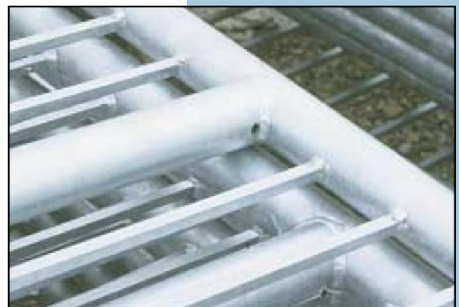
Vent holes on the outside of pipe assembly
