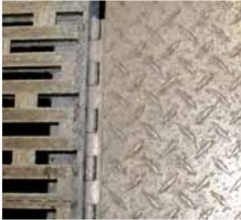
Since grating is typically used to provide multiple level flooring, quite often, grating hatches are needed to facilitate access from one level to another.
